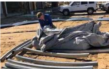
Figure 2 Edge Beam, Liner, Etc. in middle of Tank Pad
