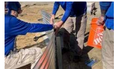
Figure 5 Forming the First Ring of Tank
