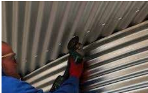
Figure 18 Using Grinder to mark the Roof
