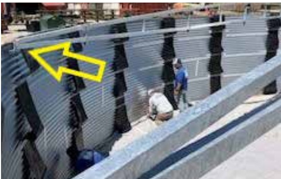
Figure 10 Shorter Truss Attached to Tank Edge Beam
